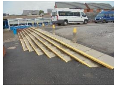
Bollards have clear markings to assist VI impaired students
