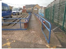
Demarcate the start and end of ramp
